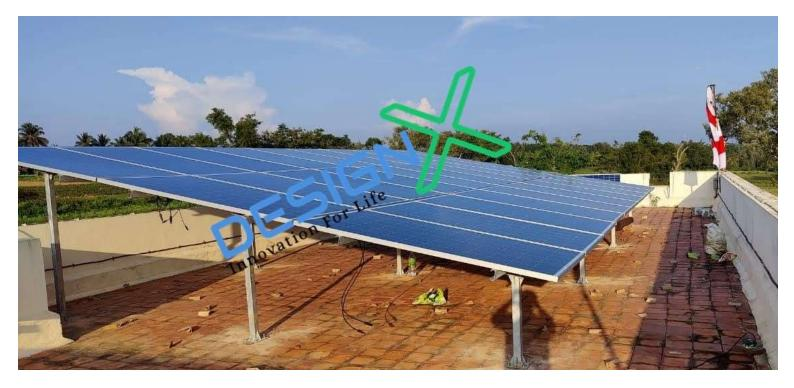
**Features:** MS 40kw MS Standard Structure with Hot Dip Galvanized Material IS 2062 HDG:60to80 MICRONS At Hassan Karnataka
